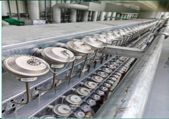
Self-diagnostic composite temperature sensor
